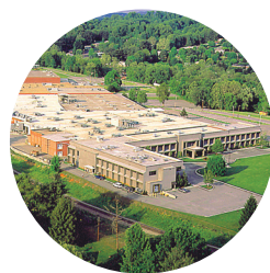
AERUS MANUFACTURING PLANT | BRISTOL, VA
